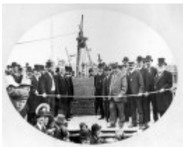
1909 - Laying of Grandstand Foundation Stone
