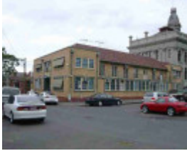
Fitzroy Police Station
