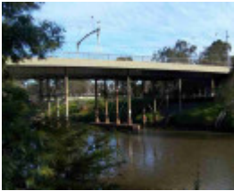
Yarra River Bridge
