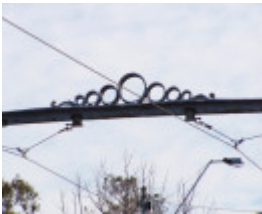
Tram poles - Swan Street
