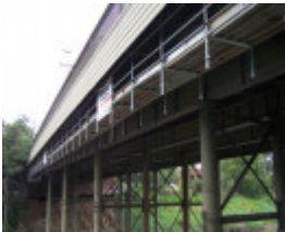
Yarra River Bridge
