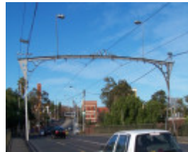
Tram poles - Swan Street
