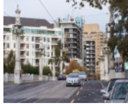
Church Street Bridge
