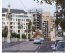
Church Street Bridge
