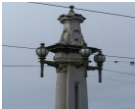
Church Street Bridge
