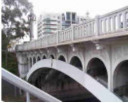
Church Street Bridge
