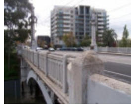
Church Street Bridge
