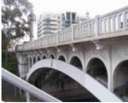
Church Street Bridge
