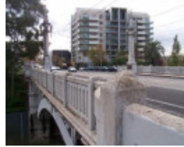
Church Street Bridge
