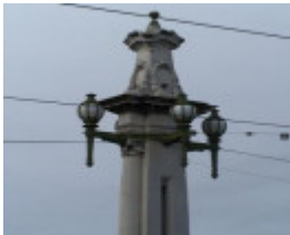
Church Street Bridge
