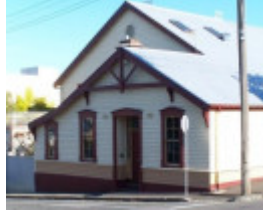
Richmond Orderly Room
