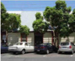
Richmond Orderly Room - 26 Gipps Street
