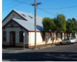
Richmond Orderly Room
