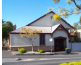
Richmond Orderly Room
