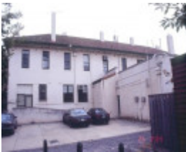
h01486 south melbourne court house and police station rear she project 2004
