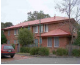
fitzroy north st georges court fitzroy north st georges court 4 unit 1-4
