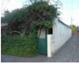
fitzroy north rowe street fitzroy north rowe street 66 unit 1
