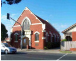
Burnley Uniting (former Presbyterian) Church
