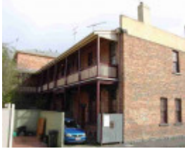
National School - 31 John Street
