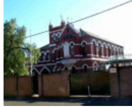
FCJ School Building
