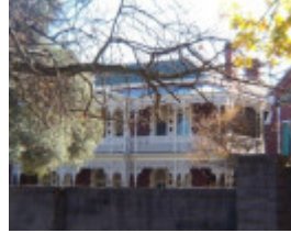
FCJ Convent Building
