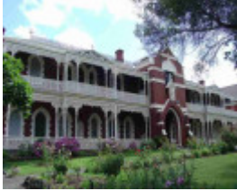
FCJ Convent Building
