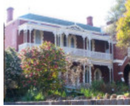
FCJ Convent Building
