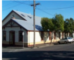
Richmond Orderly Room
