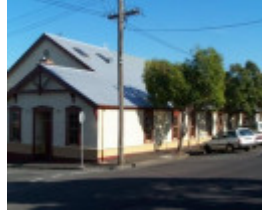
Richmond Orderly Room
