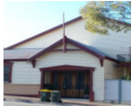
Richmond Orderly Room
