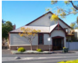
Richmond Orderly Room
