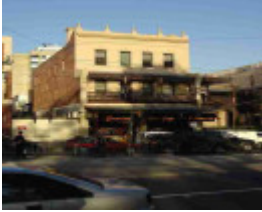
Osborne House - 44 Nicholson Street
