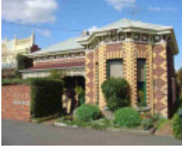
fitzroy north mckean street fitzroy north mckean street 182 unit 1-4
