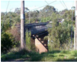
Chandler Highway Bridge
