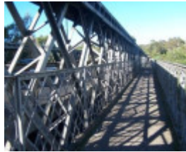
Chandler Highway Bridge
