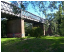
Chandler Highway Bridge
