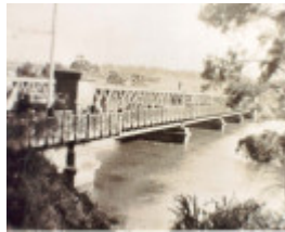
Chandler Highway Bridge - 1934
