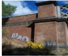
Chandler Highway Bridge
