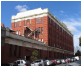
70 Oxford Street - west elevation from Oxford Street
