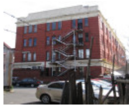
70 Oxford Street - south elevation from Peel Street
