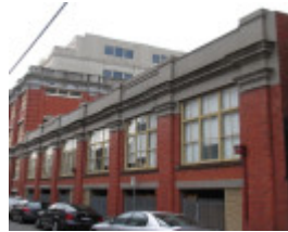
109 Oxford Street - view from Little Oxford Street
