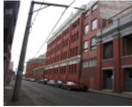
103 Oxford Street - view from Little Oxford Street
