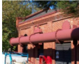
Fitzroy Gas Works Valve House
