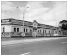
Cable Car Engine House Shed
