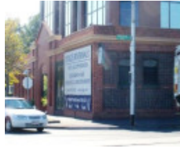
Melbourne Tramway & Omnibus Cable Tram Depot
