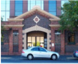
Melbourne Tramway & Omnibus Cable Tram Depot
