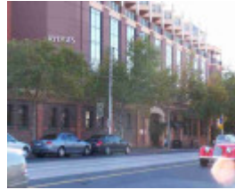
Melbourne Tramway & Omnibus Cable Tram Depot
