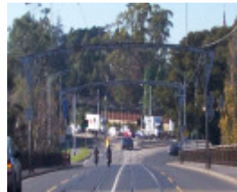
Ornamental tram poles
