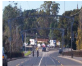
Ornamental tram poles
