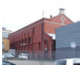
Cathedral Hall view from Young St
