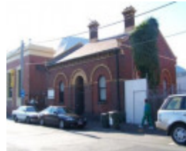
Gas Inspector's Residence
