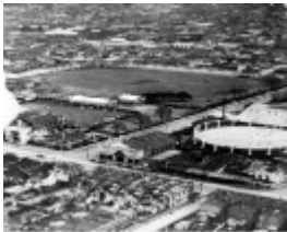
Image showing the gasometer in Gleadell Street
