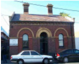
Gas Inspector's Residence
