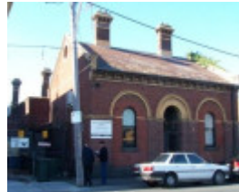
Gas Inspector's Residence
