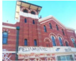
New Australian Electric Lighting Co. Power Station
