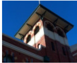
New Australian Electric Lighting Co. Power Station
