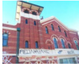
New Australian Electric Lighting Co. Power Station
