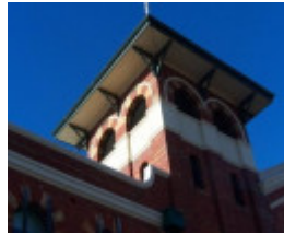
New Australian Electric Lighting Co. Power Station
