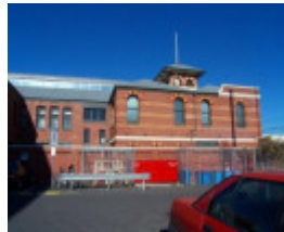
New Australian Electric Lighting Co. Power Station
