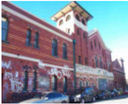
New Australian Electric Lighting Co. Power Station
