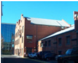
New Australian Electric Lighting Co. Power Station
