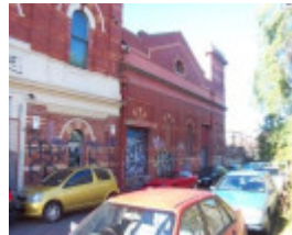
New Australian Electric Lighting Co. Power Station
