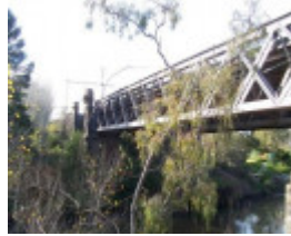
Hawthorn Railway Bridge
