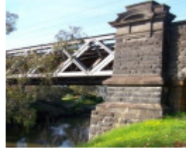
Hawthorn Railway Bridge
