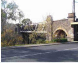
Hawthorn Railway Bridge
