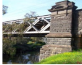
Hawthorn Railway Bridge
