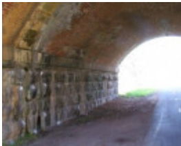
Hawthorn Railway Bridge
