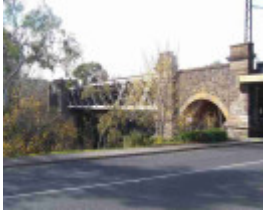
Hawthorn Railway Bridge
