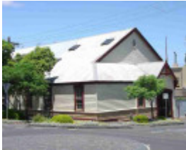
Richmond Orderly Room - 24 Gipps Street
