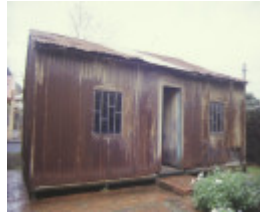
Abercrombie House 399 Coventry St Sth Melbourne Abercrombie Rear View Jul 1999
