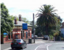
West Richmond Railway Station
