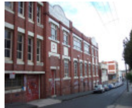
Collingwood Perry St rear 35 johnston St.JPG
