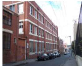
Collingwood Perry St rear 35 johnston St.JPG
