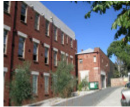
Rear of 45 Victoria.JPG
