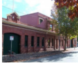
Cable Tram Engine House
