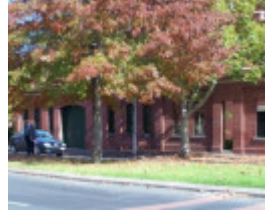
Cable Tram Engine House
