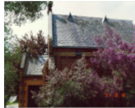
Uniting Church Main Rd Eltham Colour 2- Shire of Eltham Heritage Study 1992
