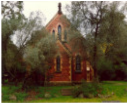
Uniting Church Main Rd Eltham Colour 1 - Shire of Eltham Heritage Study 1992
