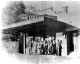
207 - JN Burgoyne 820 Main Rd Eltham 03 - This shop photographed after the south side addition was completed (ELHPC No. 702) - Shire of Eltham Heritage Study 1992
