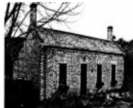
211 - Shillinglaw Cottage Main Rd Eltham 03 - Shire of Eltham Heritage Study 1992
