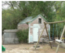
Former Harvey Farmhouse, 2000 Hamilton Highway, Murgheboluc
