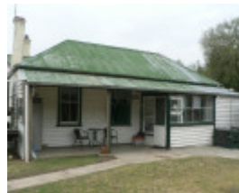
Former Harvey Farmhouse, 2000 Hamilton Highway, Murgheboluc
