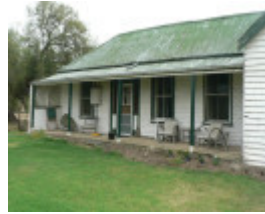
Former Harvey Farmhouse, 2000 Hamilton Highway, Murgheboluc
