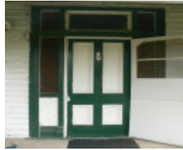
Former Harvey Farmhouse, 2000 Hamilton Highway, Murgheboluc
