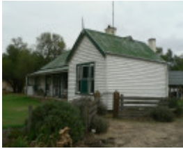
Former Harvey Farmhouse, 2000 Hamilton Highway, Murgheboluc
