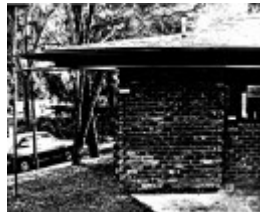
221 - Eltham South Kindergarden 03 - Shire of Eltham Heritage Study 1992
