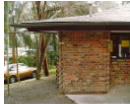
Eltham South Kindergarden Colour 1 - Shire of Eltham Heritage Study 1992
