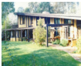
Pittard Residence 430 Mt Pleasant Rd Colour 2 - Shire of Eltham Heritage Study 1992
