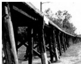
Railway Timber Trestle Bridge, Panther Place
