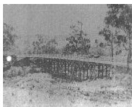
Railway Timber Trestle Bridge, Panther Place - PREVIOUS MAIN ROAD BRIDGE OVER DIAMOND CREEK AT ELTHAM - ALSO A TIMBER TRESTLE BRIDGE
