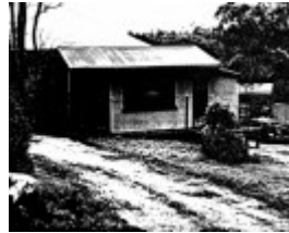
241 - Alan Marshall Bungalow Eltham - Shire of Eltham Heritage Study 1992
