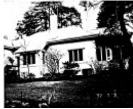
244 - Stanhope House Eltham 03 - Shire of Eltham Heritage Study 1992
