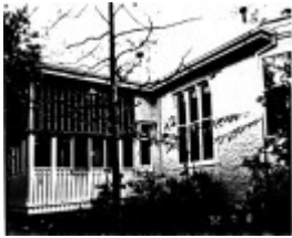
244 - Stanhope House Eltham 04 - Shire of Eltham Heritage Study 1992
