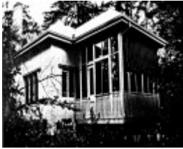
244 - Stanhope House Eltham - Shire of Eltham Heritage Study 1992
