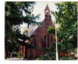
St Margaret's Anglican Church Eltham Colour 1 - Shire of Eltham Heritage Study 1992
