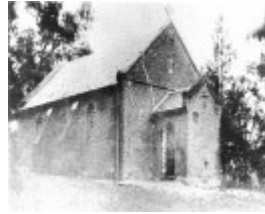
247 - St Margaret's Anglican Church Eltham 17 - Demolished Eltham Catholic Church (ELHPC No. 681) - Shire of Eltham Heritage Study 1992
