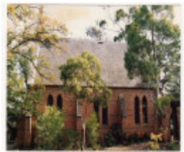
St Margaret's Anglican Church Eltham Colour 2 - Shire of Eltham Heritage Study 1992
