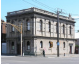
FORMER FREEMASONS HALL SOHE 2008
