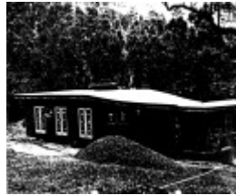
261 - The Busst House Eltham 04 - South elevation photographed during construction - Note the curved eastern end and roof following the descent of the stair within - Shire of Eltham Heritage Study 1992
