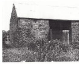
Former Bateman House Black & White 1 - Shire of Eltham Heritage Study 1992
