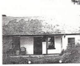
Former Bateman House Black & White 3 - Shire of Eltham Heritage Study 1992
