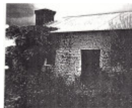
Former Bateman House Black & White 2 - Shire of Eltham Heritage Study 1992
