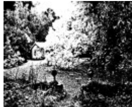
268 - Sweeneys Cottage Eltham 18 - Shire of Eltham Heritage Study 1992
