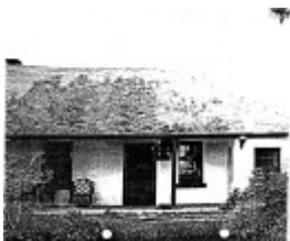
268 - Sweeneys Cottage Eltham - Shire of Eltham Heritage Study 1992
