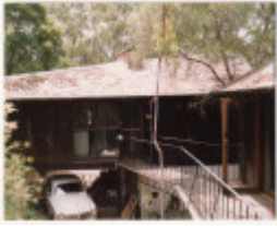
Downing Le Gallienne Residence Eltham Colour 5 - Shire of Eltham Heritage Study 1992
