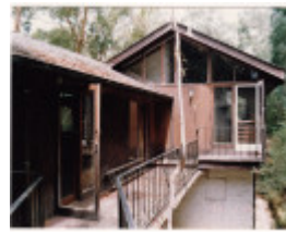
Downing Le Gallienne Residence Eltham Colour 4 - Shire of Eltham Heritage Study 1992
