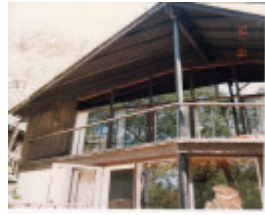
Downing Le Gallienne Residence Eltham Colour 2 - Shire of Eltham Heritage Study 1992
