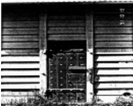
277 - Portable Timber Lock Up Eltham 04 - Shire of Eltham Heritage Study 1992
