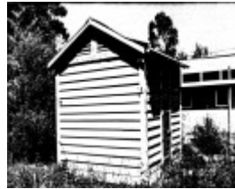
277 - Portable Timber Lock Up Eltham 02 - Shire of Eltham Heritage Study 1992
