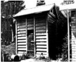
277 - Portable Timber Lock Up Eltham - Shire of Eltham Heritage Study 1992
