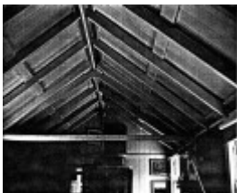
278 - Hurstbridge Railway Station Building 07 - Shire of Eltham Heritage Study 1992
