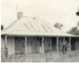
B1302 Cottage- Hume Hwy, Avenel
