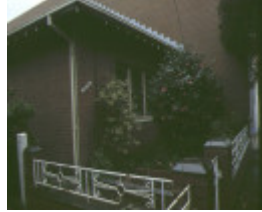
108 116 gladstone street south melbourne iron fence
